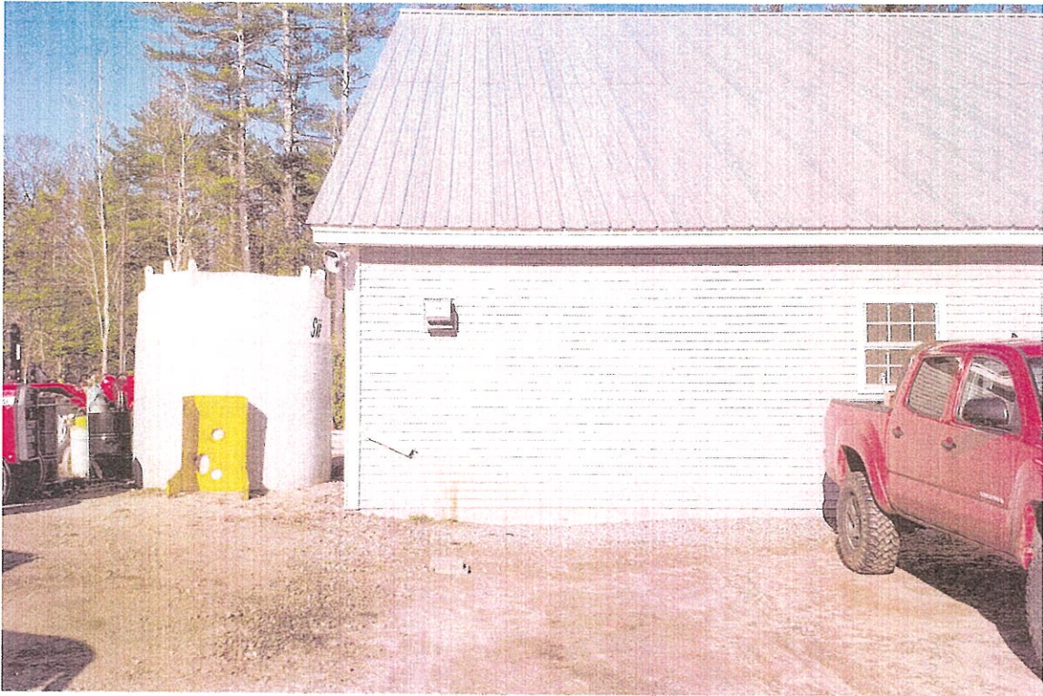
Back side of Building
