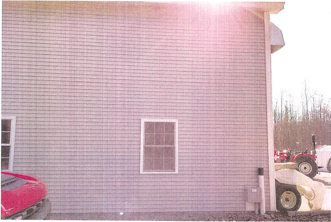
High way side of Building
